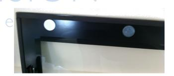
A fixing magnet is screwed into the frame to align with metal attractors fixed to the top of the mirror.
